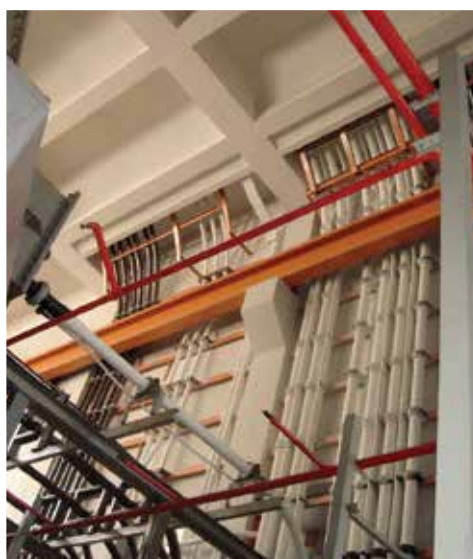
Electrical cables coated with PROMASTOP® CIS at a warehouse (below) in Ayer Rajah, Singapore.
