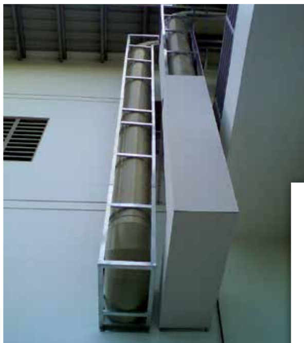
General M&E services enclosure at the carpark of Tseung Kwan O residential building in Sai Kung District, New Territories, Hong Kong (above) and outside the warehouse of 9 Benoi Sector, Singapore (left). Both use PROMATECT®-H boards.
