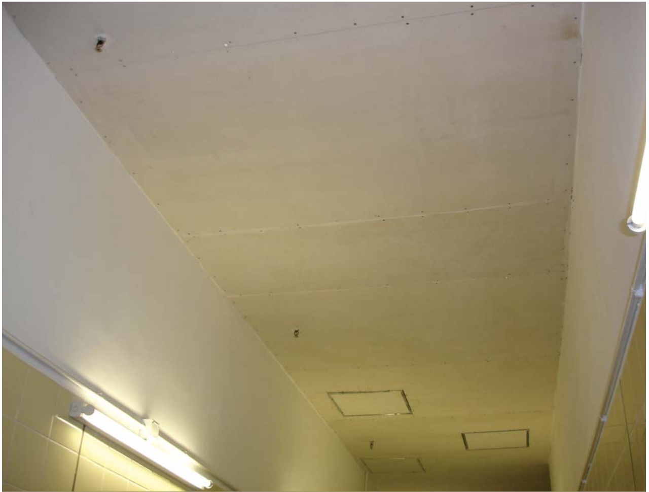
Opposite PROMATECT®-H integrity only suspended membrane ceiling at Hospital Pantai Ayer Keroh, Malacca, Malaysia.
